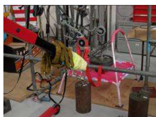
The weight being removed after testing
